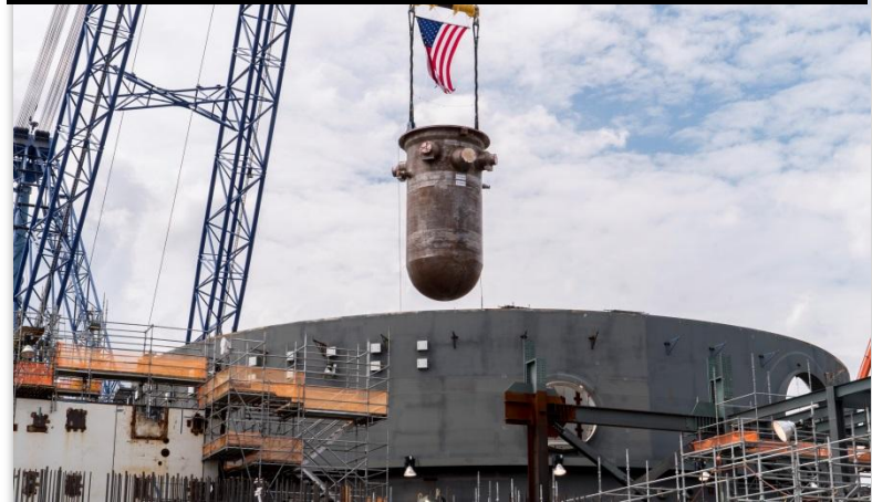
Unit 2 Reactor Vessel Placement – August 2016
