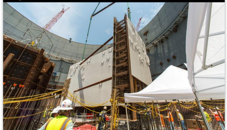
Vogtle Unit 4 CA05 Module Placement – June 2016
