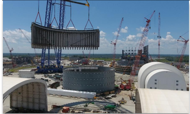
Unit 2 CA03 Module Placement – July 2016
